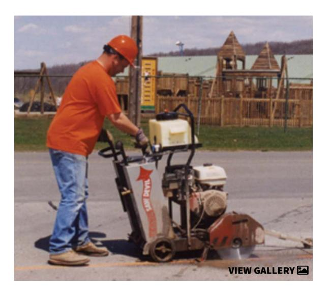
Walk-behind concrete saws come in a range of sizes, from compact 4- or 5-hp electric-powered models up to large, diesel-powered pavement saws boasting 65 hp or more. Determining which size will be most productive for a particular cutting task largely comes down to the length and depth of the cut, and the material your customers will be cutting.
